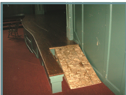
Hazardous Narrow Ramp
